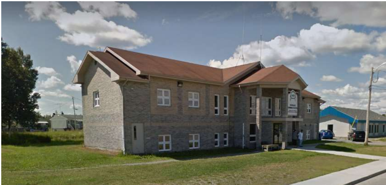
Figure 4 – Administration Offices at Lac Simon First Nation Community, Quebec
