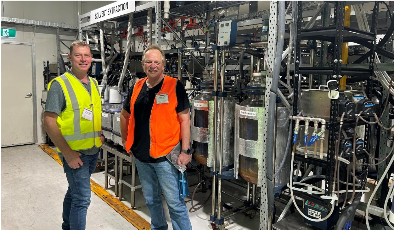
Figure 1 – Haydn Daxter and Dr. Nigel Brand at Nagrom the Mineral Processor’s Pilot Plant
